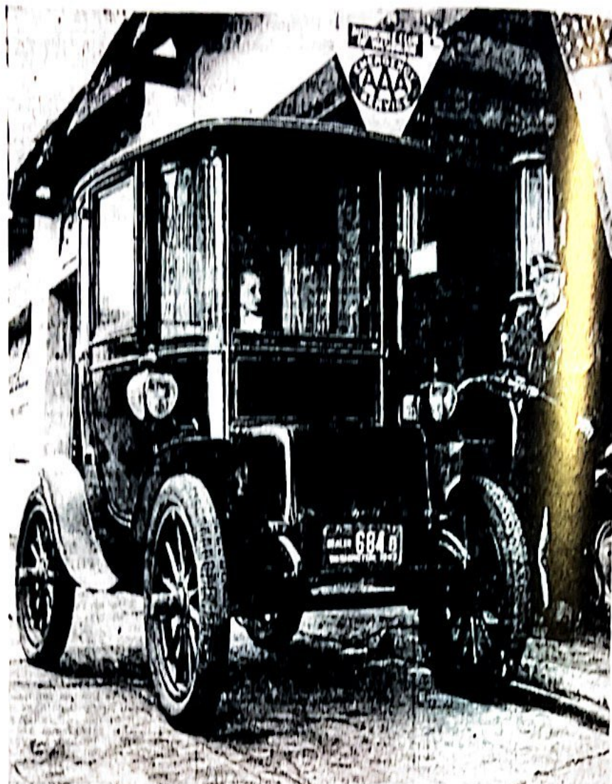
Get Up and Go —It'll run, gas or no gas, says Garageman Crist Keffler about this gas ration defying 1911 Baker Electric, owned by Miss Mave Olds of 55 Broadway. Run by batteries at a safe, sane and law abiding 20 miles an hour, it may be no thing of streamlined beauty but will get you there—if not too far away, when your A coupons are gone.
